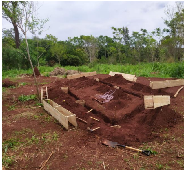
Figure 13 – IMAD’s initial 6x3 m rhomboid office space receives its foundations.
